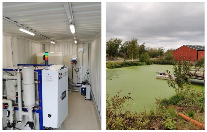
Figure 1: Left – Aquarden containerized PFAS pre-treatment system comprising chemical flocculation and microfiltration. Right – Pond polluted with PFAS from firefighting activities. Note the green algae plume that can interfere with the PFAS adsorption process if not properly removed by pre-treatment systems.
